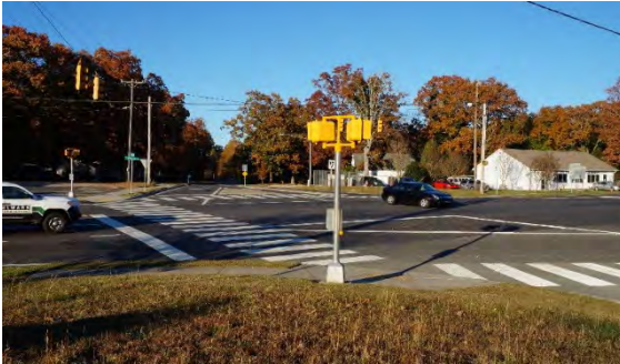
Marked crosswalk and pedestrian signal heads at Faucette Mill Road
