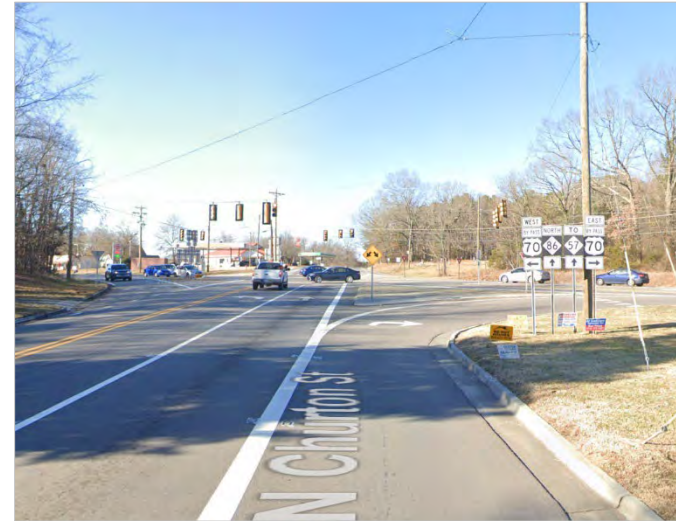
NC 86 / Churton Street at US 70 – looking north
