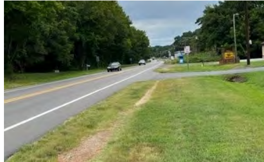
Worn path observed west of US 70 Business (Churton Street)
